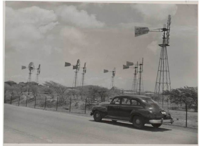
Figure 10. Windmill-powered abstraction wells near Julianadorp , Curaçao ( Nationaal Archief ).
