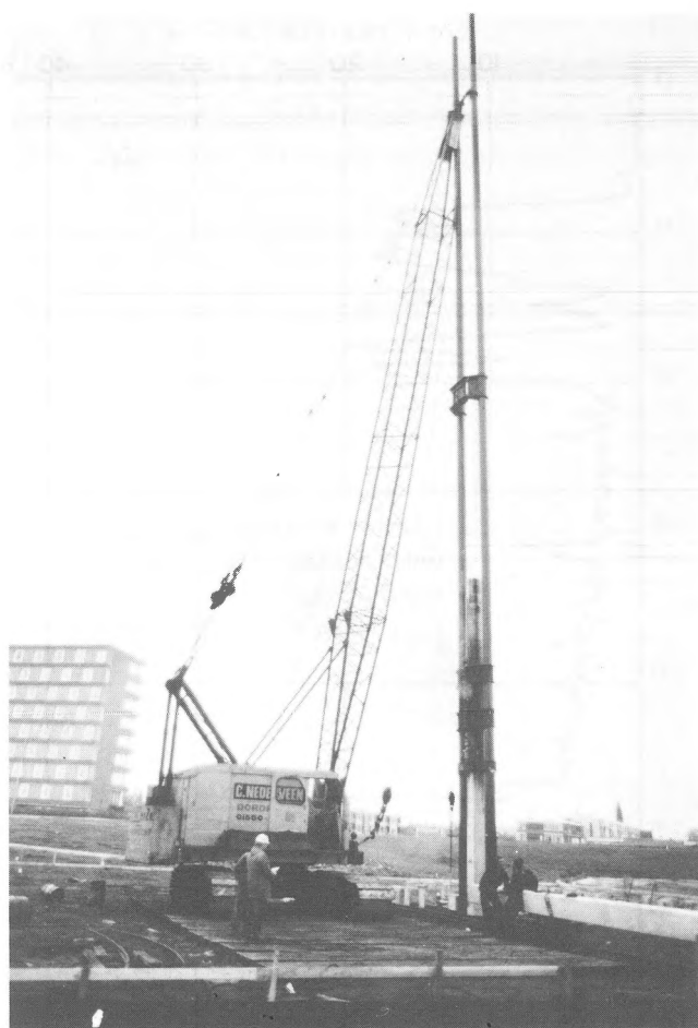
Fig. 5 Driving of precast concrete piles.
