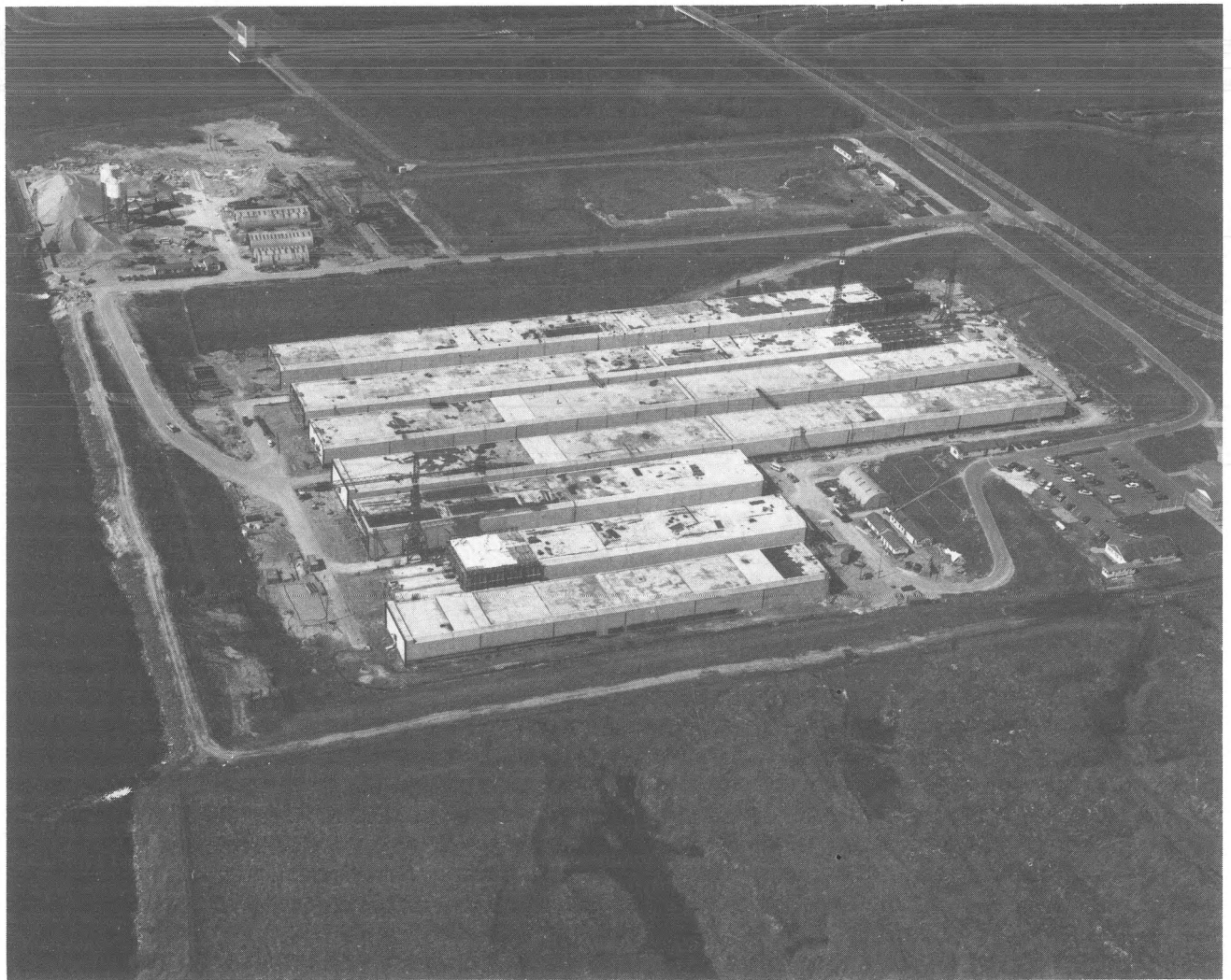
Fig. 9. The Amsterdam Noord dry dock with the immersion tunnel units of the Hem railway tunnel.
