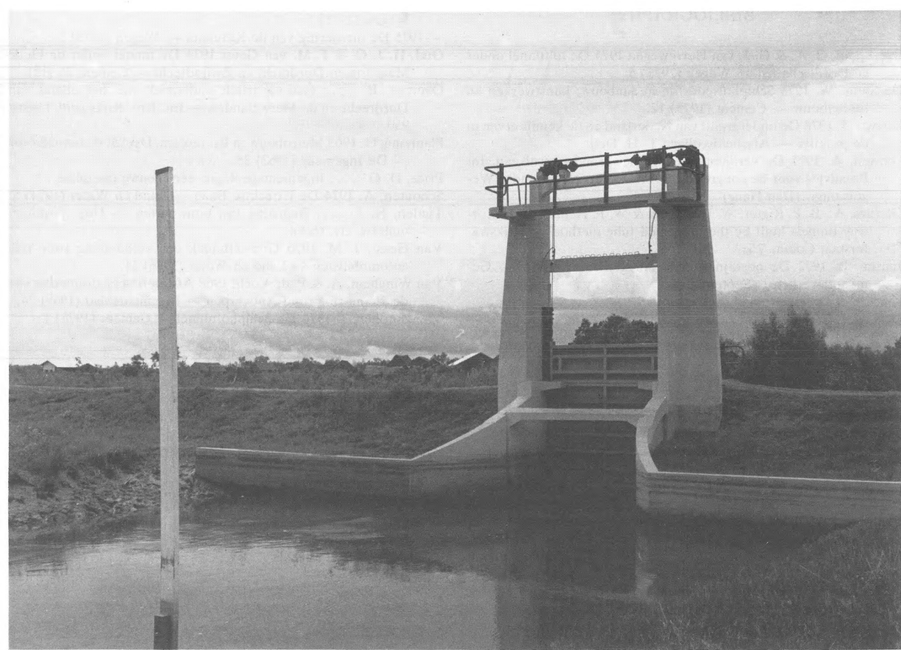
Plate III Modern drainage sluice for removal at low tide of excess water from low-lying coastal polders in Malaysia (Tanjong Jurong). The light-weight gates consist of aluminium.
