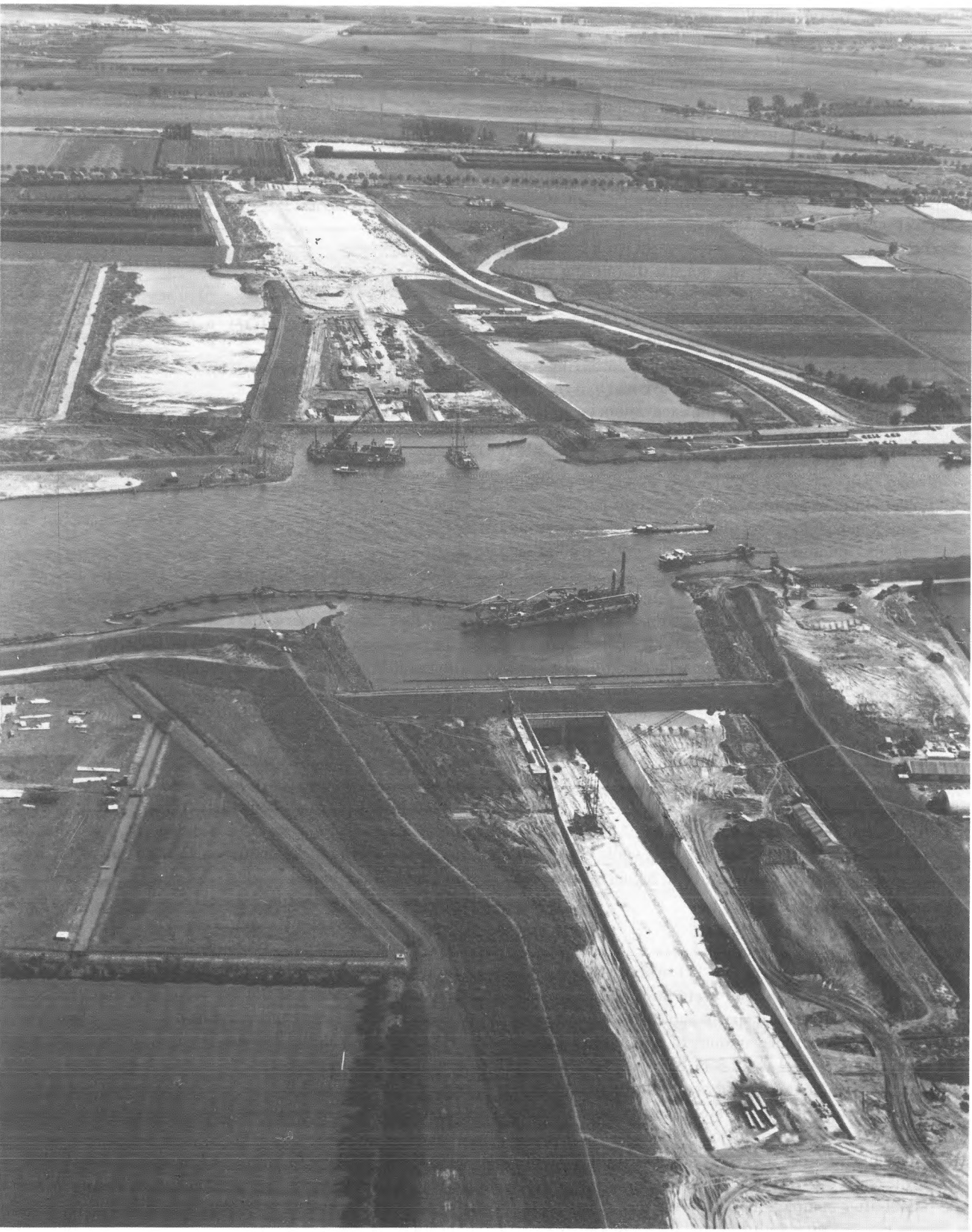
Fig. 15 The Gouwe aquaduct on the A-12 highway, under construction.
