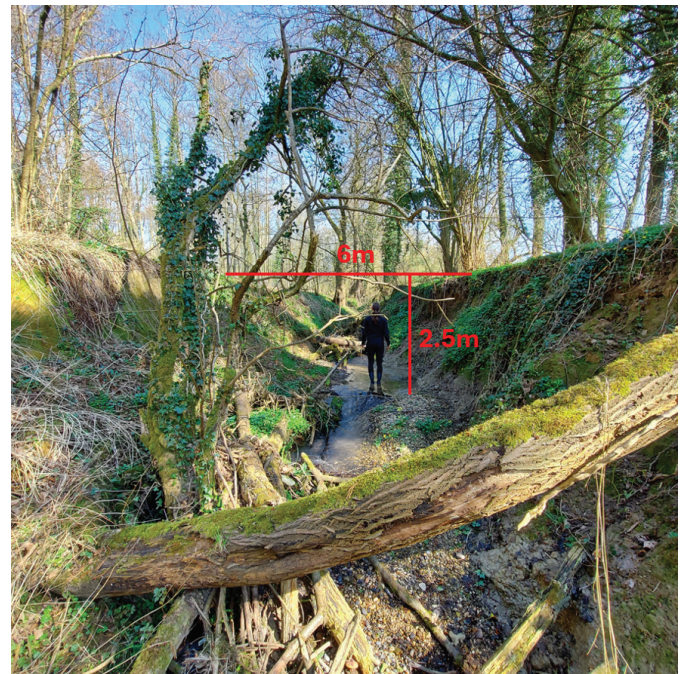
Figure 2. Heavily eroded brook bed in the Dutch region of the Noor brook. Fluvial erosion has deepened and widened the brook considerably over the last decades due to (1) landscape evolution during average discharge and (2) landscape revolution during short intensive peak discharges. It is estimated that approximately 2 m of the depth is due to erosion and 0.5 m is related to microtopography (floodplain aggradation). In the front, some degraded remains of a woody debris jam are visible. The gravel underneath the wood debris was artificially added as armouring layer to avoid deep scours.
