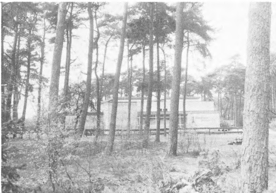
Fig. 23 The pumping station of "Beerschoten".
