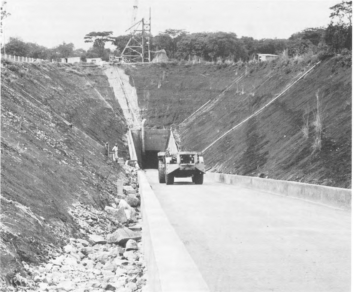
Photo 1 An Eimco T20 truck on the Baluba main service incline.
