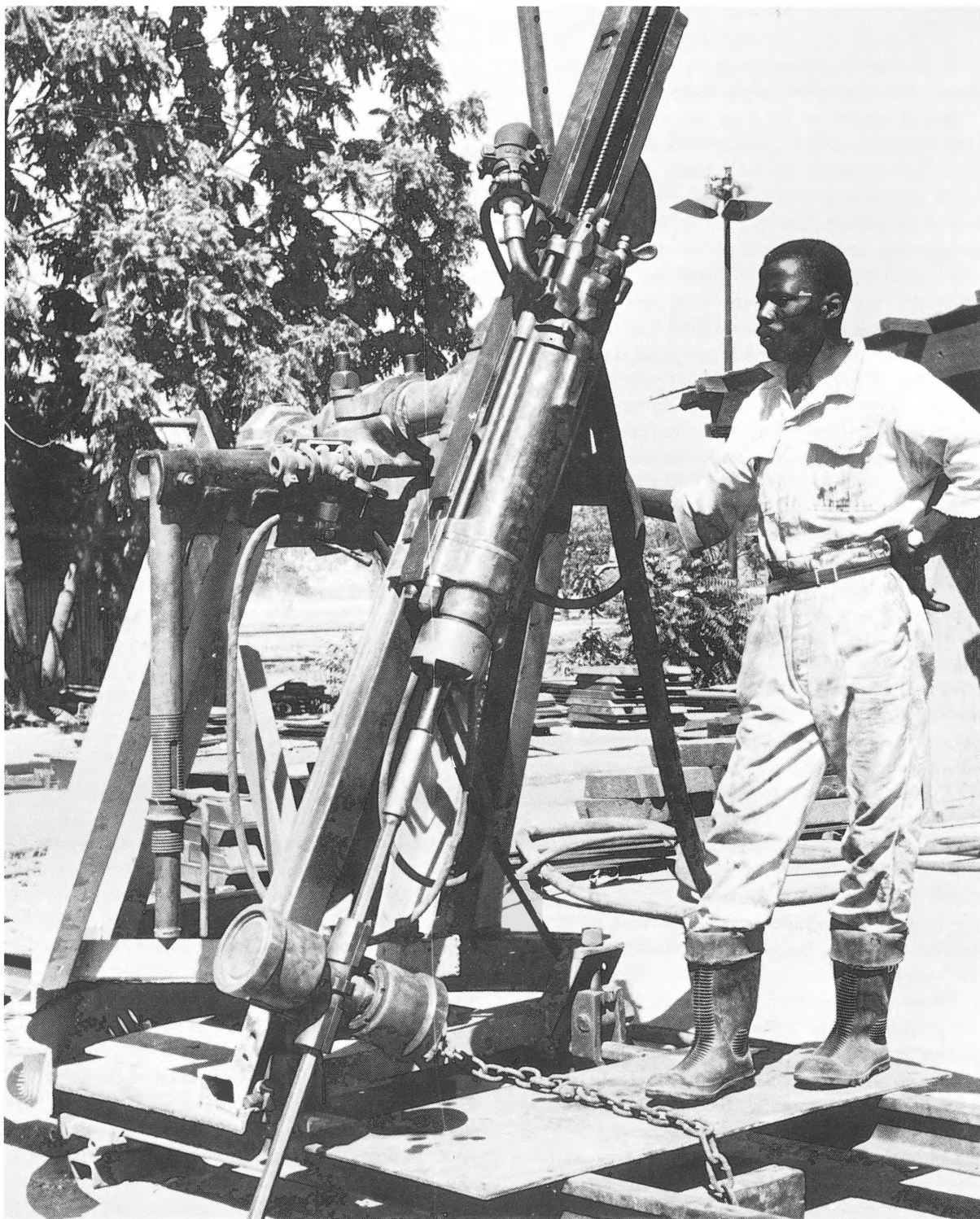
Photo 2 A Gardner Denver stope drifter, skid drill rig.
