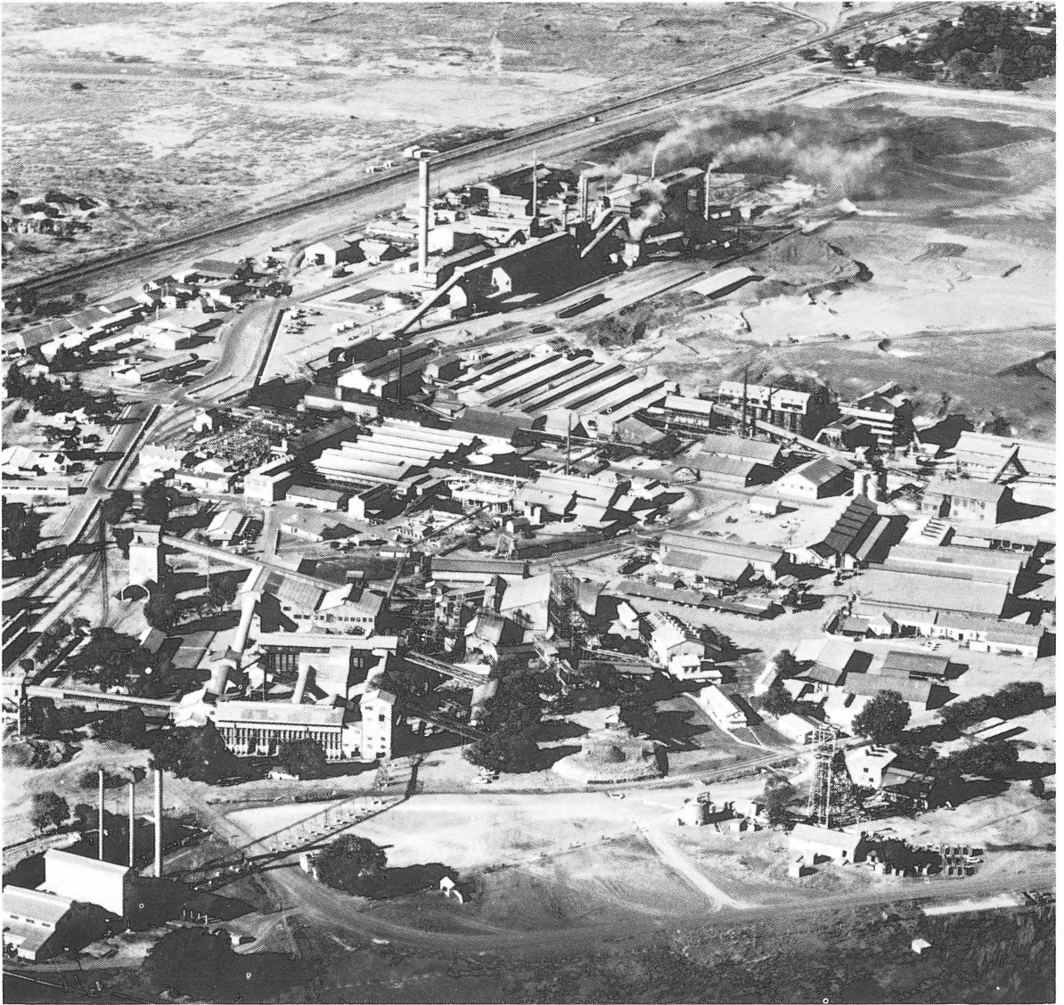
Photo 1 An aerial view of the metallurgical plants.
