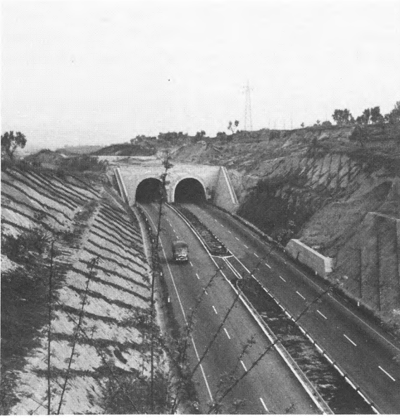
Fig. 15 Roofed gallery to protect autostrada from sliding masses of head scarp.
